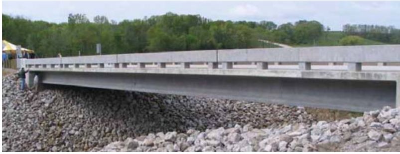
Fig. 6: First UHPC Bridge Constructed in the United States (in Iowa), Source: [1]
