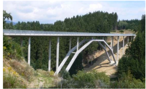
Fig. 20: UHPC bridge in Austria, Source: [10]
