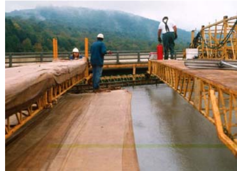
Fig. 8: Curing of UHPC Bridge Deck Source: [8]
