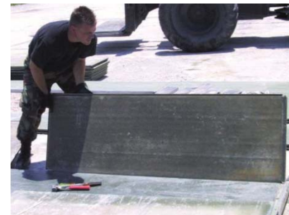
Fig 4: AM-2 matting requires a 16-person team to deploy [13]
